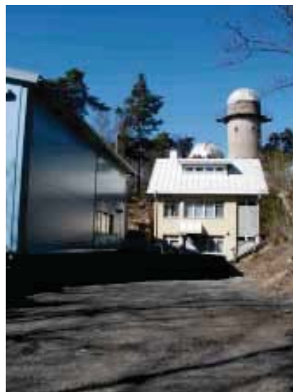
Figure 4-3: Opteon polishing facilities
